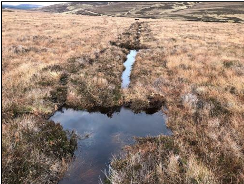
Plate 2.1 Example of peat dams to be used for on-site drain blocking.
