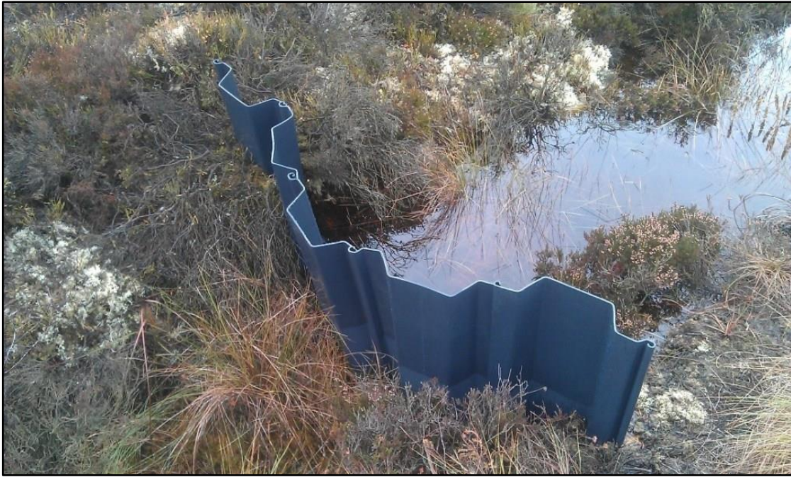
Plate 2.2 Example of plastic dams to be used for on-site drain blocking.
